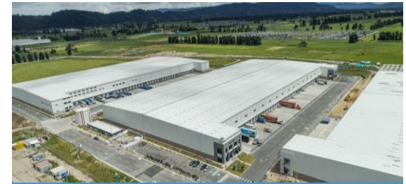
Logistic Park Calle 80, Bogotá, Colombia
